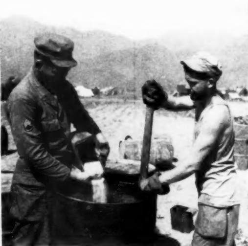
Into each 55 gallons of gasoline approximately 14 pounds of napalm are poured. Lacking a mechanical mixer, a wooden paddle serves the purpose.
